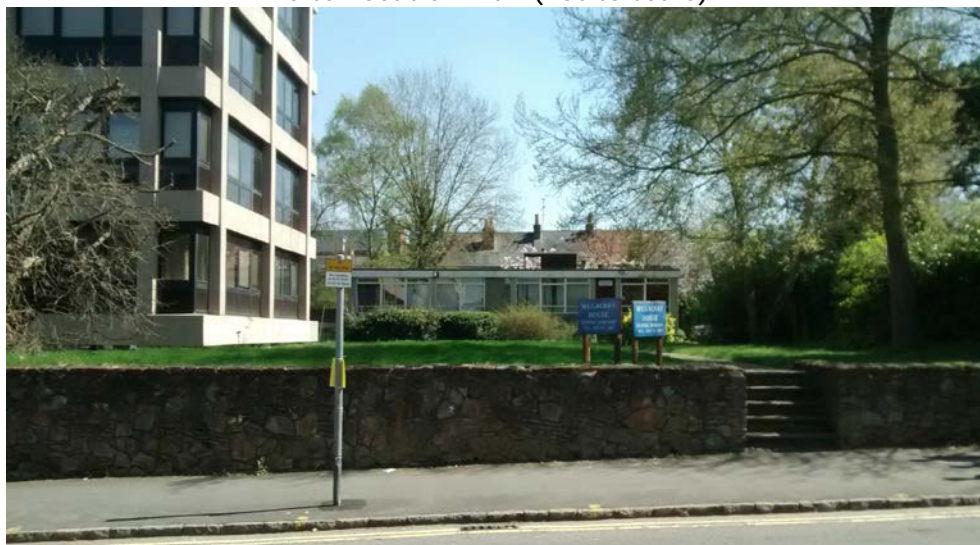
Site photograph from Eldon Road
