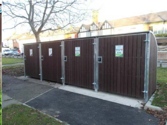
Proposed bin storage (the proposed units will only consist of two of these).
